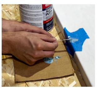
Apply Bondo\* on the damaged area Leave enough material to be able to shape the area. Remove the tape before curing.
