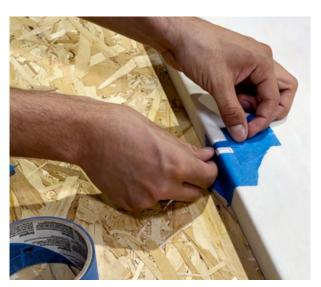
Apply tape keeping a clearance of 1/16" offset from the repair area.
