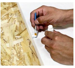
Paint must be applied within 10 minutes of mixing. Allow paint to dry for a minimum of 6 hours, before use.
