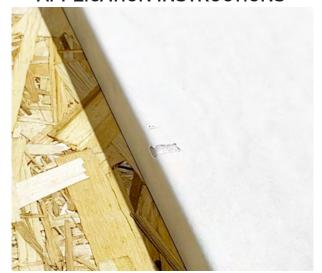
Remove broken or loose pieces from damage area.
