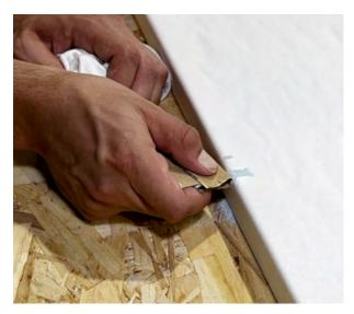
Sand excess bondo\* following the shape of the area. Clean the area with alcohol before proceeding with paint.
